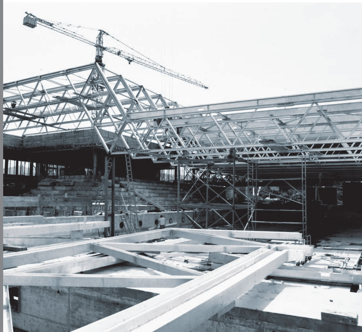
Hallenbad West in Freiburg-Mooswald
